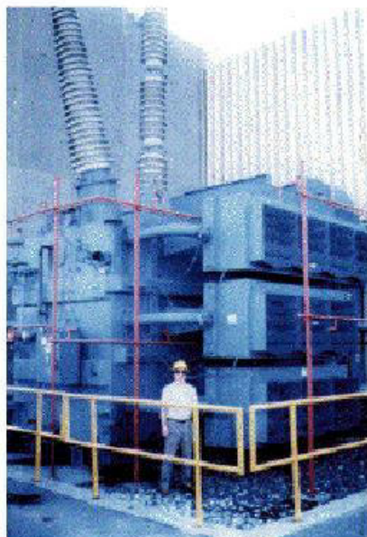
PJM Public Service Step Up Transformer
