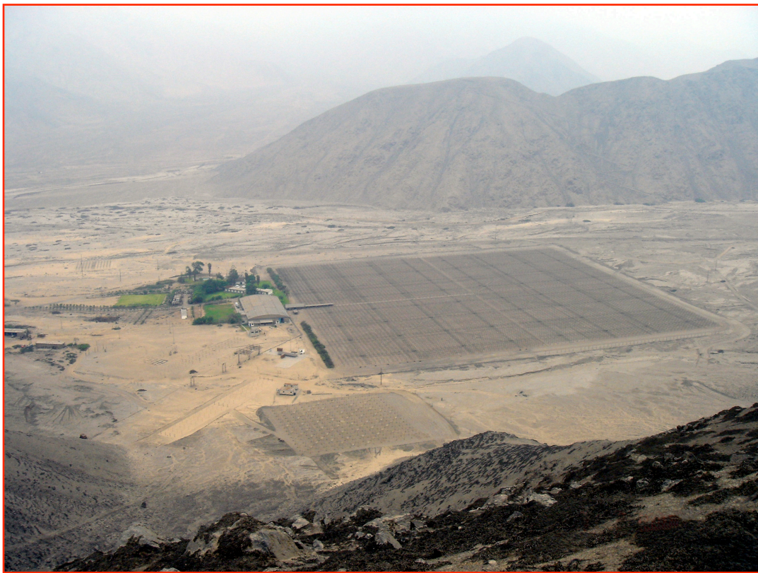
Jicamarca: the first phased array incoherent scatter radar observing the lowest magnetic latitude. Photo: Koki Chao
