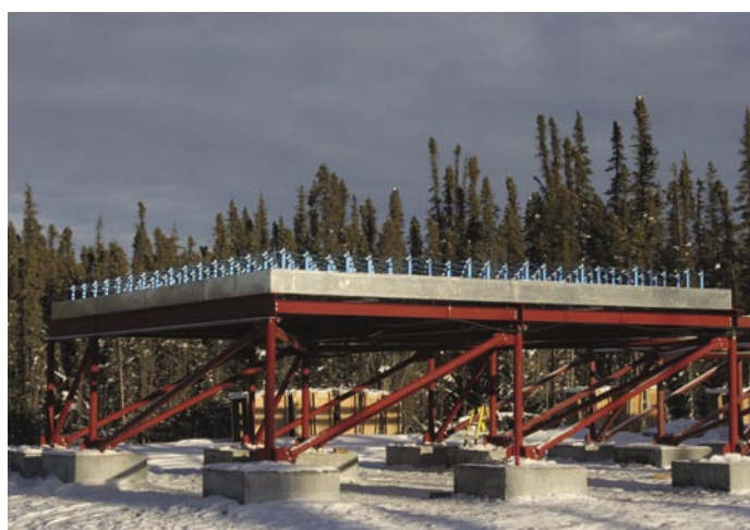
Approximately square array at HAARP.
