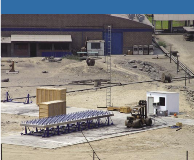
AMISR array and calibration antennas at Jicamarca.
