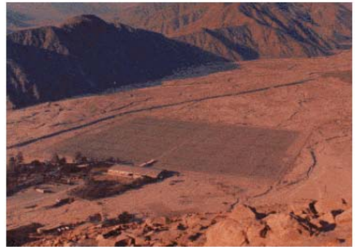
Jicamarca Radar at 49.9 MHz uses 18,432 dipoles
