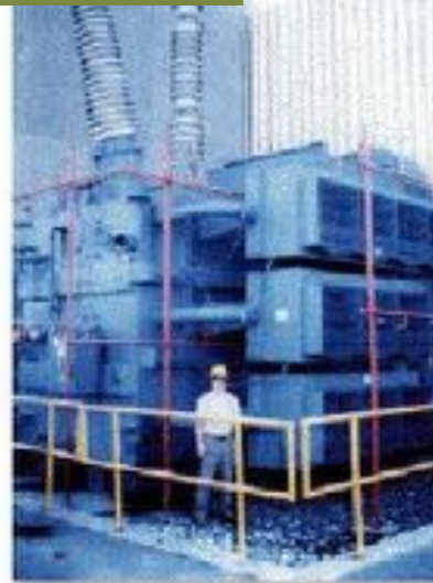
A large space storm in 1989 caused currents which damaged this transformer and shut off power for six million people for nine hours.
